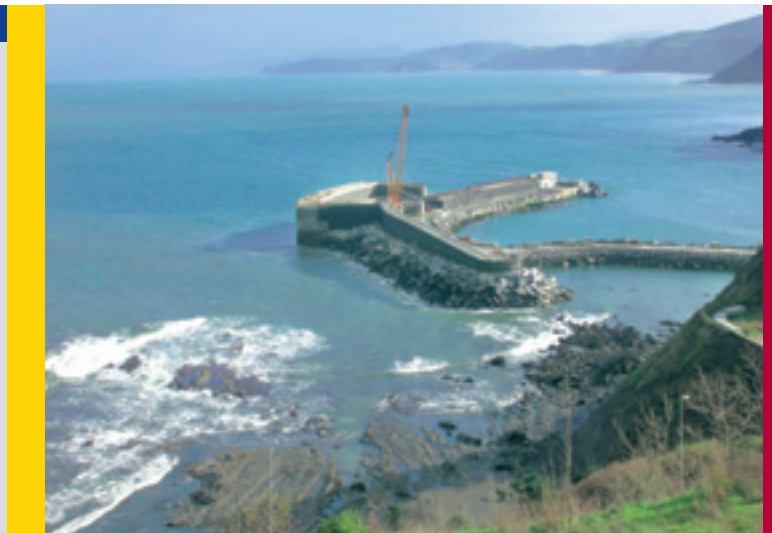
Mutriku breakwater wave power station during construction
